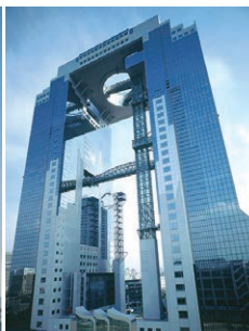
Umeda Sky Building (Japan)
